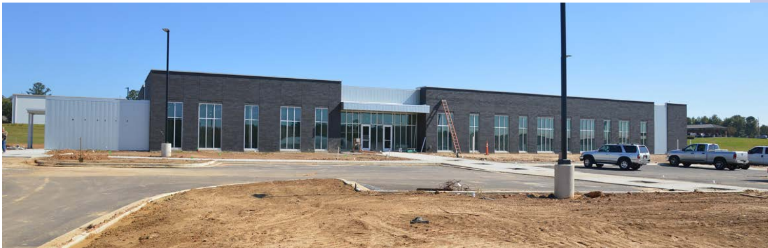
Progress on the new CMPDD office building currently under construction.
