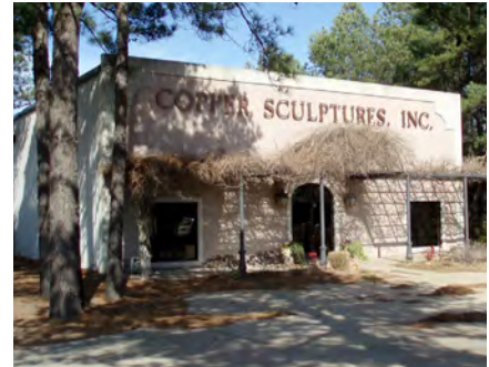
The RIF grant was used to construct road improvements along Lakeland Drive adjacent to Copper Sculptures, improving traffic flow and access to this and other businesses along the roadway.
