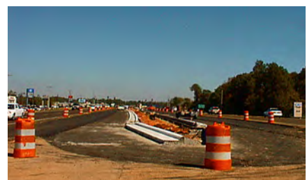
Widening of Lakeland Drive in Flowood.
