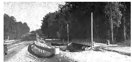
Construction of the Reservoir Bikeway/ Pedestrian Trail.
