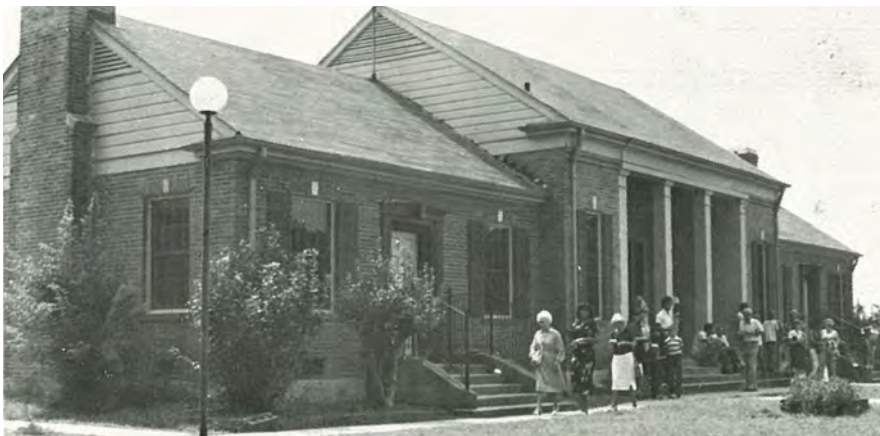
CMPDD and the Mississippi Council on Aging assisted Magee in obtaining funds to renovate its Community Center to create a multi-purpose Senior Center.
