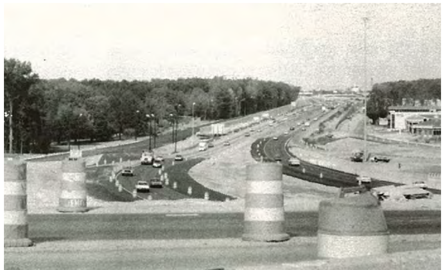
Work in progress on Interstate 55 between Meadowbrook Road and Lakeland Drive.
