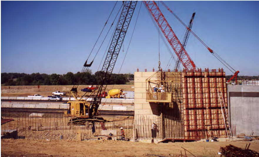
Construction on the interchange at I-55 and MS Highway 463 in Madison.
