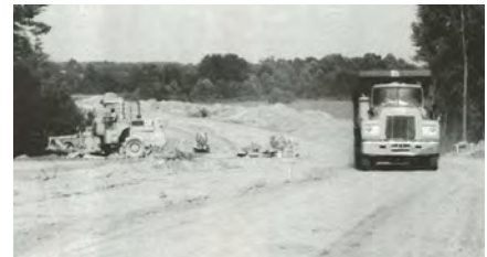
Construction of the Highland Colony Parkway in Madison County.
