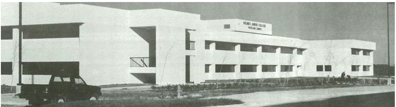
Diligent efforts by CMPDD and Ridgeland officials resulted in Ridgeland being the first Mississippi City ever to receive funding approval under the Secretary's Discretionary Fund, Department of HUD, for water and sewer lines for the High Technology Branch of Holmes Community College.
