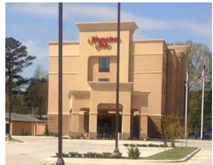
Hampton Inn in Richland, funded with a CMDC loan.
