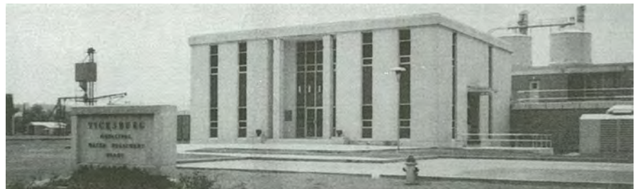
The District obtained EDA funds used in the construction of a new water treatment facility in Vicksburg.
