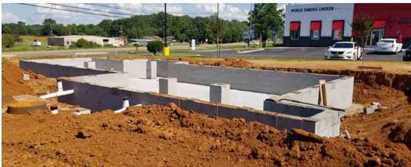
Construction of Checkers Restaurant in Pontotoc, MS
